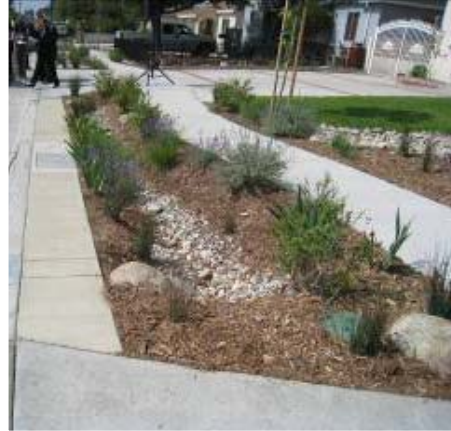
Photo of retrofitted public easement at Elmer Avenue decentralized Stormwater Management Project.
