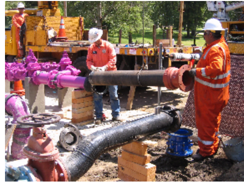
31,800 feet of purple pipe has been installed since 2006.
