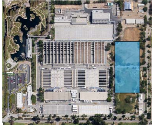
Location of the added wastewater facilities at D.C. Tillman Water
