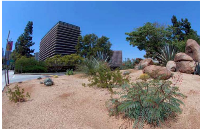
The LADWP Ferraro Building displays California-friendly landscape that uses less water than traditional lawns.
