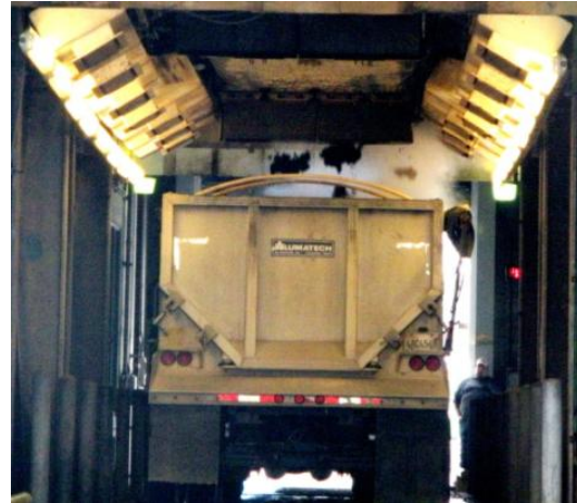
Existing Truck Loading Facility at HTP
