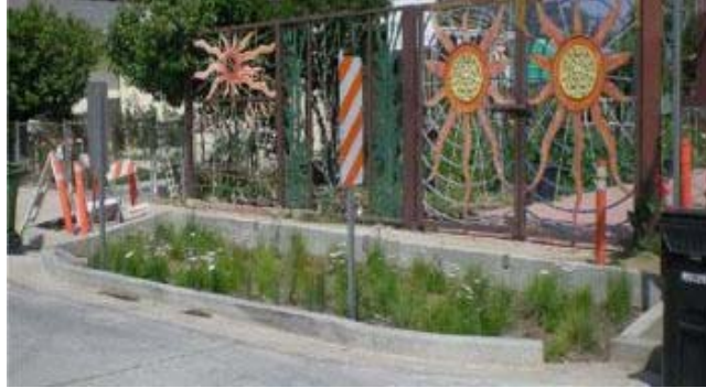
The Riverdale Green Street Project utilizes stormwater parkway planters to treat and infiltrate polluted urban runoff.
