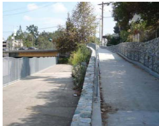
Pedestrian bridge crossing Los Angeles River at Taylor Yard.
